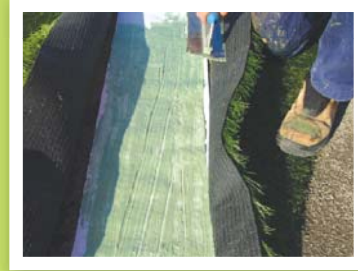
Trowelling adhesive onto seaming tape
