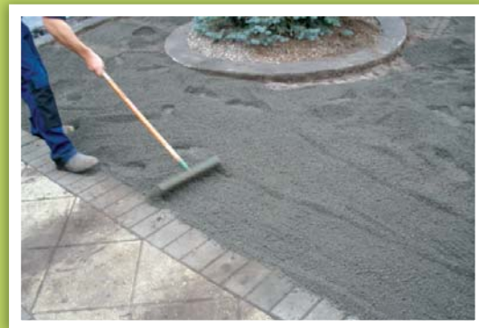
Spreading the 20mm crushed rock
