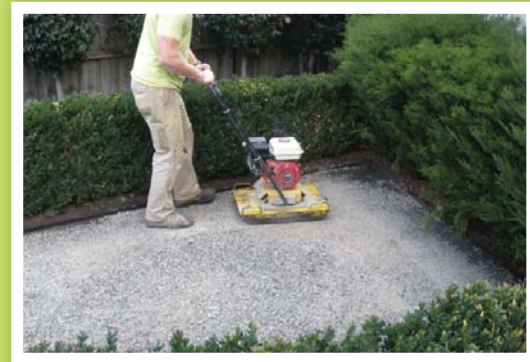
Compacting the base
