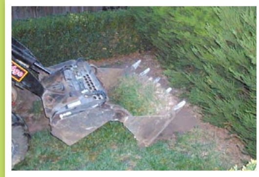
Excavation of area by hand or machine
