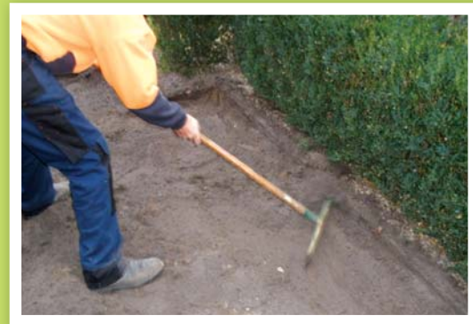
Allow for grass height when installing next to edges
