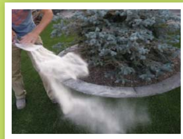
Broadcasting the infill sand
