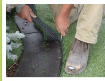
Trimming around edges
